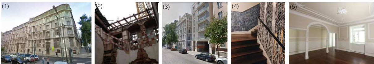
Figure 4 - (1) Main façade, before the intervention. (2) Ceiling collapse, before intervention. (3) Rua Luciano Cordeiro Facade, after intervention. (4) Main stair core, after intervention. (5) Interior Room, after intervention.
