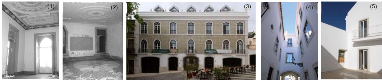
Figure 1 - (1) Interior main room, before the intervention. (2) Main entrance atrium, before the intervention. (3) Main Façade, after the intervention. (4) Rua das Damas, after rehabilitation. (5) Outdoor patio, after intervention.
