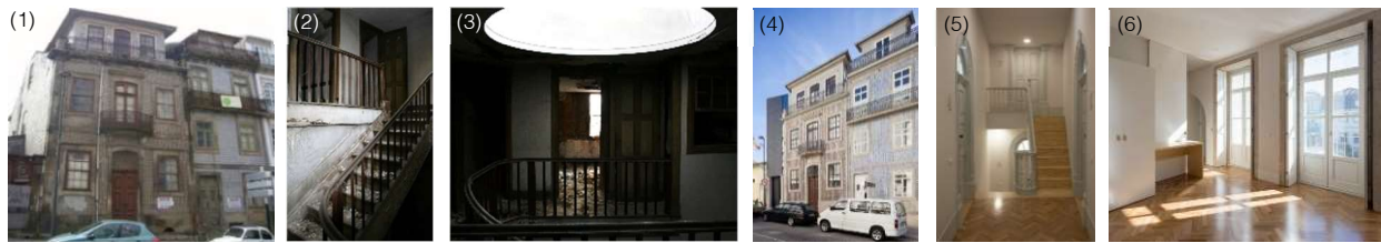
Figure 3 - (1) Main facades, before the intervention. (2) Stair core, before the intervention. (3). Skylight, before the intervention. (4) Main facades, after intervention. (5) Stairs no. 432, after the intervention. (6) Interior Room, after intervention.
