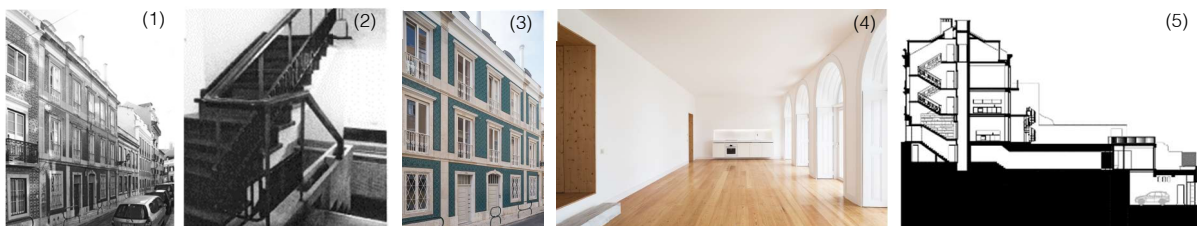
Figure 2 - (1) Main façade, before intervention. (2) Main stair core, before intervention. (3) Main façade, after intervention. (4) Main room, after intervention. (5) Section, after intervention.
